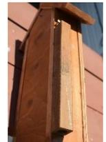
11. Once the mount is fastened, the side can be put on the house. The sides are fastened to the back of the face, not along-side. With the sides fastened to the face, the roof and bottom are fastened.
