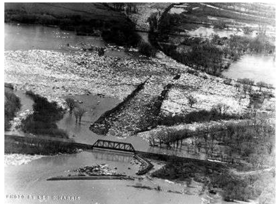
Mandan, Railroad Bridge over the flooded Heart River in 1943. (Submitted by Russel Kruger)
