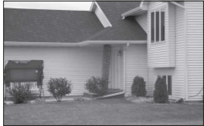
Figure 25. Porch problems due to shrink and swell.
