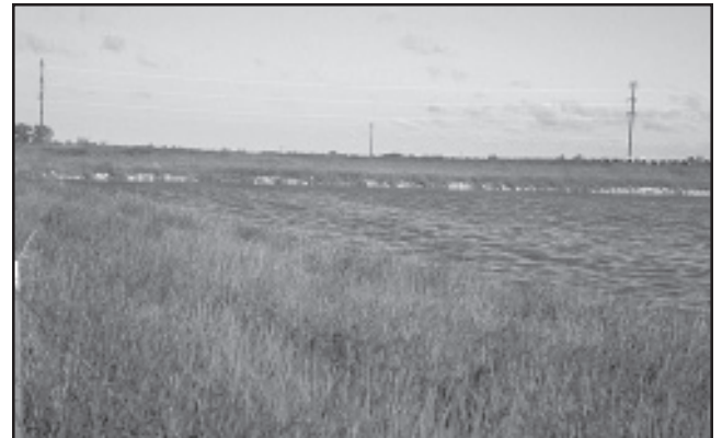
Figure 24. Sewage lagoon, West Fargo.
