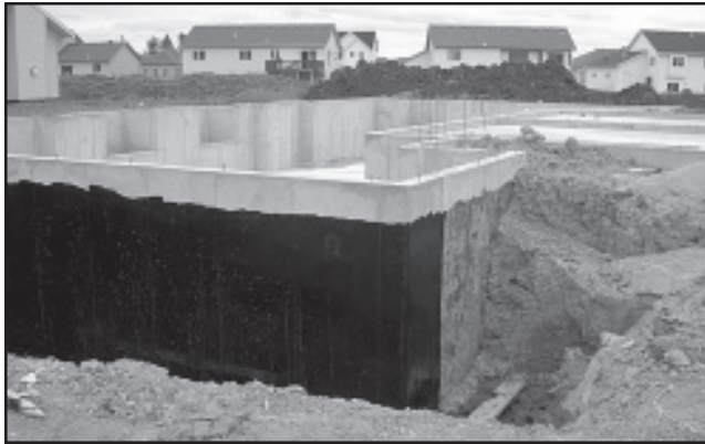
Figure 22. Concrete basement construction.
