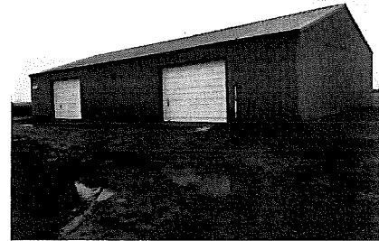
The main departmental field storage shed is small and dated. Doors are 9 feet high so limit size of equipment that can be stored.
